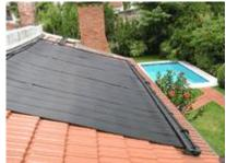
The size of the system is calculated according to the size of the swimming pool, the placement of installation and the distance from the solar panels to the pump.
